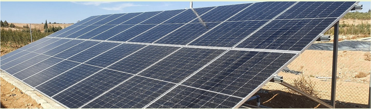
Figure 1. 22-kWp solar PV on-grid ground-mounted system for farm of Saleh Afash in Al-Achaari.
