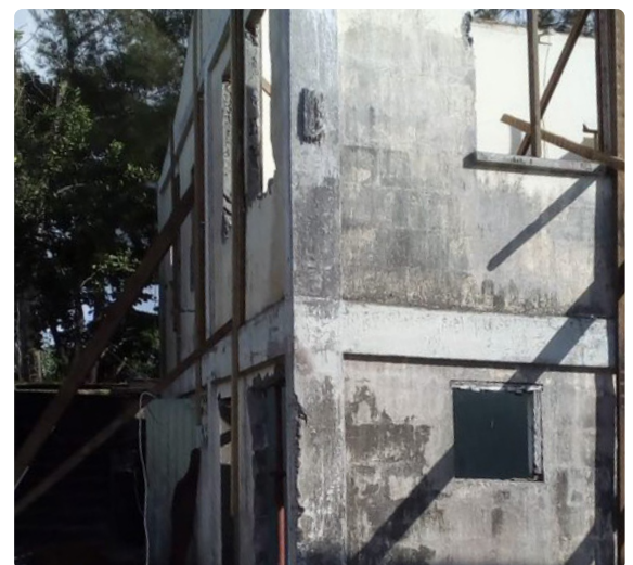
The Centre before reconstruction. ©UNICEF
