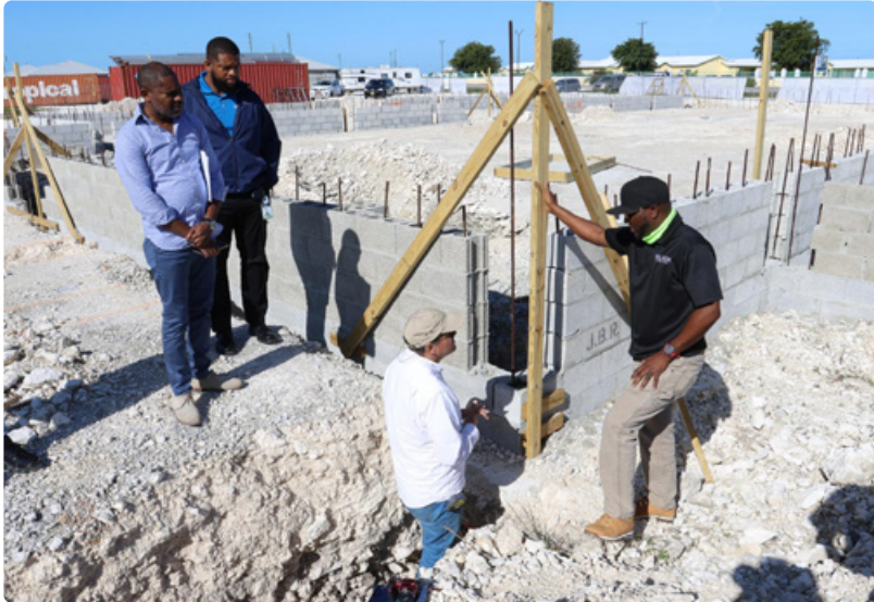
Constructing hurricane-resilient shelters on the Abaco islands. ©UNDP
