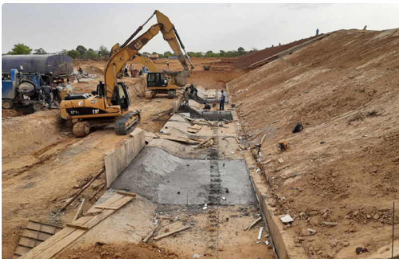
Work in progress on the Niangdo Dam Project. ©UNDP
