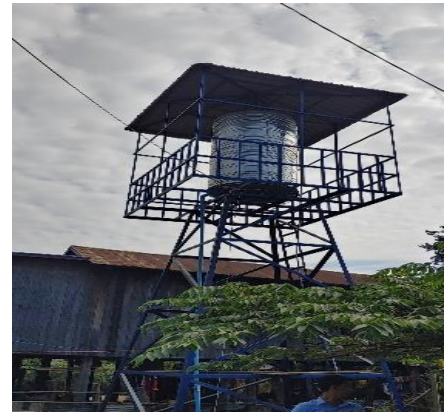
Photo 2: Installed water tank facility in the community
